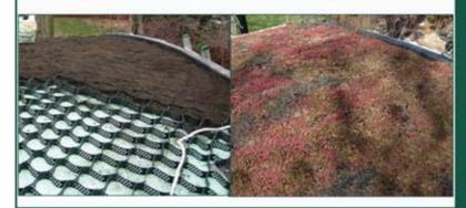
LSG Series® and SlopeGrid® cellular confinement systems consist of a giant blanket of 3-D connected cells forming a honeycomb like blanket. The system keeps soil in place making a suitable environment for plants to grow and thrive.
