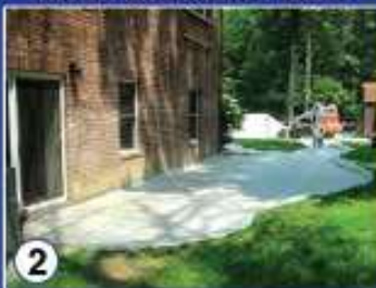
Install Geotextile Fabric
