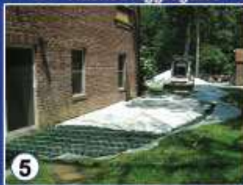
Infill Grid With 3/4" Washed Aggregates
