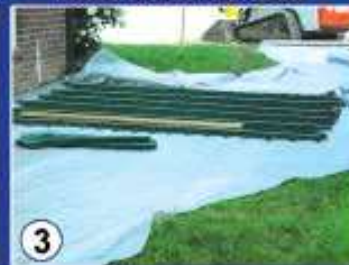
Install Stabilizer Grid
