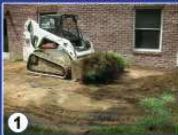
Excavate Job Site
