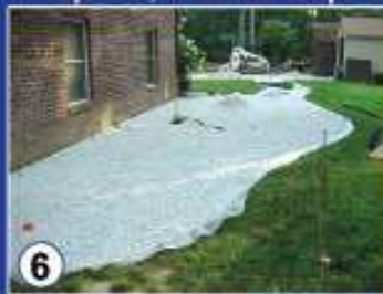
Spread, Level & Tamp
