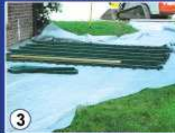
Install Stabilizer Grid
