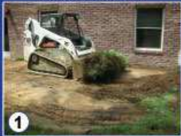
Excavate Job Site
