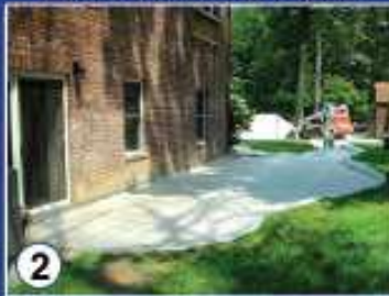
Install Geotextile Fabric
