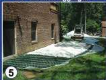
Wash Stones And Allow To Completely Dry. Mix Stones With Gravel-Lok In A Cement Mixer Or Wheelbarrow
