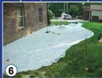
Wash Stones And Allow To Completely Dry. Mix Stones With Gravel-Lok In A Cement Mixer Or Wheelbarrow
