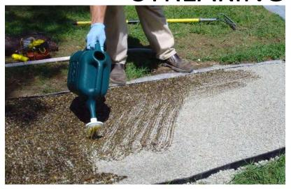
When applying Gravel-Lok with a watering can it can be difficult to regulate the flow. Keep it moving and sprinkle lightly. See photo below that shows "streaking" as a result of applying too much liquid in certain areas.
