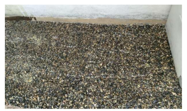
If too much liquid is applied, foaming will occur. In some cases, you can crush the foam with a brush. This must be done immediately and will only work if there is a small amount of foaming.
