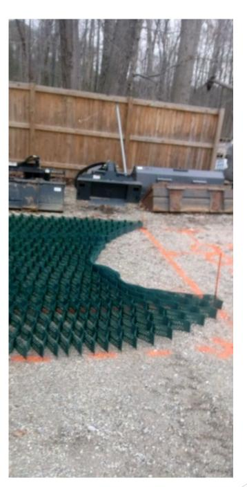
Go to center of grid at 11.25' (on 22.5' length side) and stake those cells out at the perimeter.
