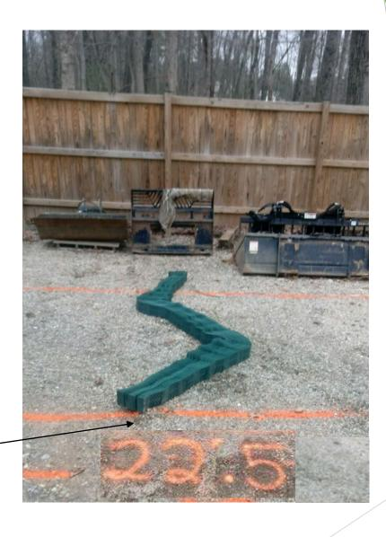
Attach the four corner cells of the grid to the four corner stakes. The grid will resemble an 'hourglass' shape.
