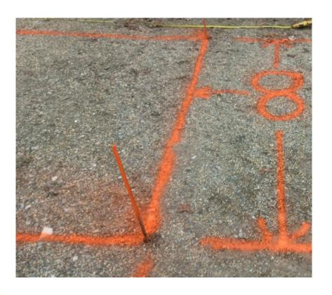
After measuring and placing all four stakes at the corners, lay the grid bundle in the center, around the 11.25' mark (on 22.5' long side)
