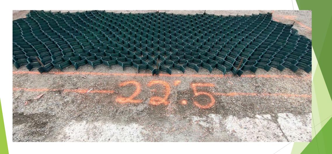
Apply the same technique to the shorter sides. First start in the middle at about the 5<sup>th</sup> or 6th cell (4' to the center)
